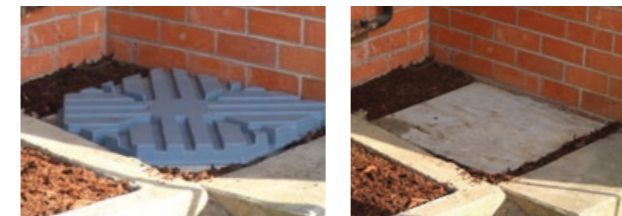
Figure 1: Concrete or heavy duty plastic slabs to be placed under the storage tank.
